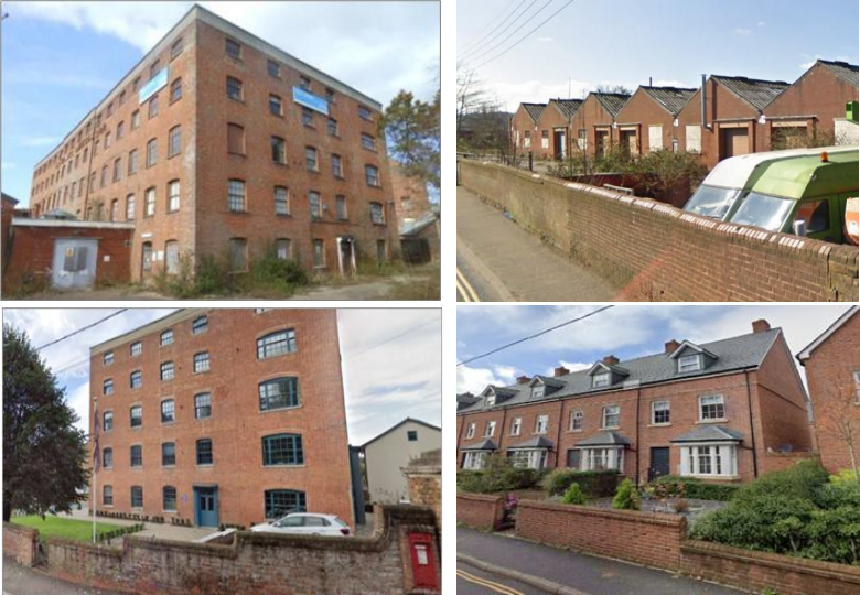
Example: Otter Mill, Switchgear factory (left) and site (right), Ottery St Mary in 2013 and 2022
