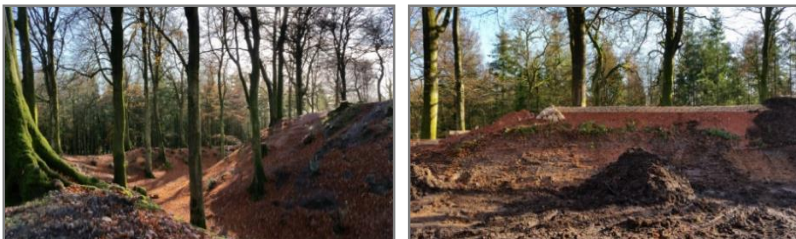
Woodbury Castle restoration project 2017- 2018, Woodbury Common.
